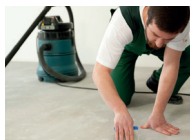
Cut off the tongue in the boards to be installed in the first row.
