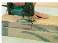
Cut off the tongue in the boards to be installed in the first row.
